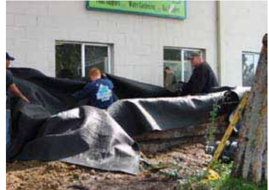
Monterey Project, installation of liner Image courtesy Aquascape, Inc.
