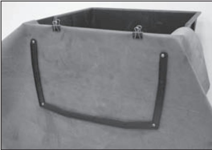
Fig. 24 Drape the liner over the front of the skimmer and attach it using the spring clips and check that the liner is smooth across the face of the skimmer.
