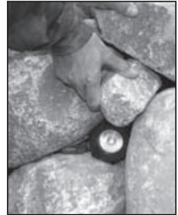
Fig. 30 Set your underwater lights in between your boulders so they are hidden from view.
