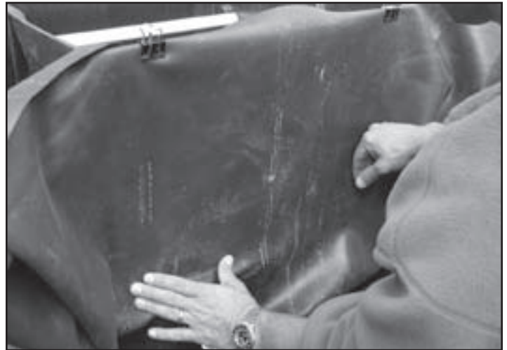
Fig. 12 Place the liner against skimmer and hold in place with the supplied clips.
