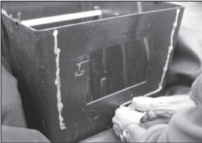
Fig. 11 Apply a bead of Silicone to the face of the skimmer.
