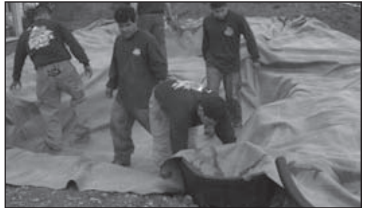
Fig. 9 Place the liner on top of the underlayment following the same installation procedures. Make sure liner is positioned in such a way that allows it to extend and completely cover the opening of the skimmer.
