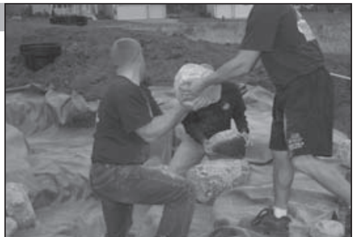
Fig. 28 Starting at the bottom, set the largest character boulders first then fill in with the smaller ones.
