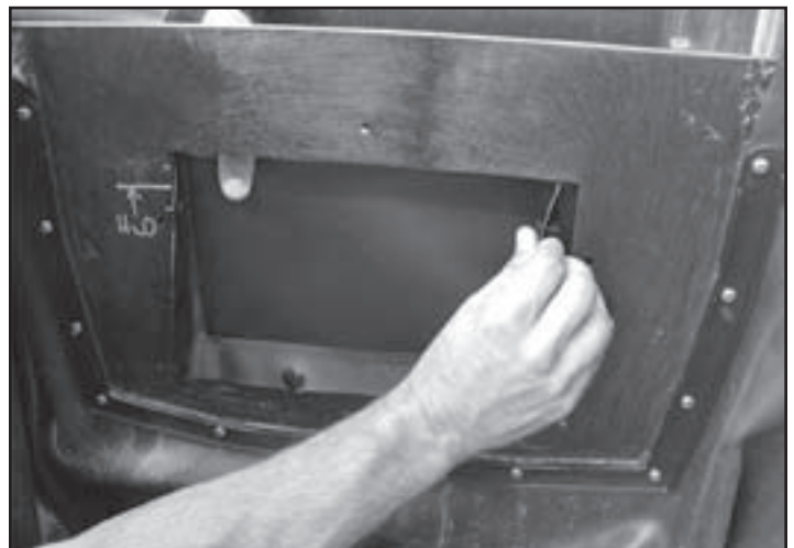
Fig. 20 Pull the bellows flap through the skimmer opening and secure to the skimmer with the fasteners.
