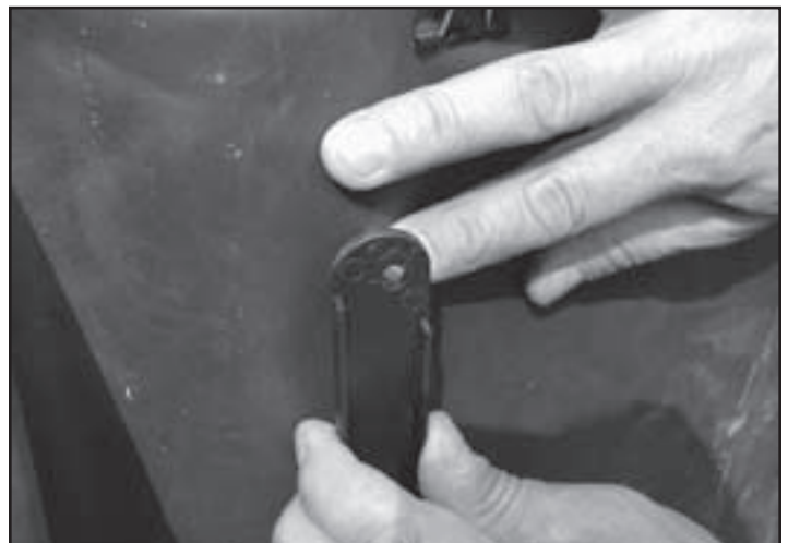
Fig. 14 Start at the “U” frame and using an awl as a guide start your first screw.
