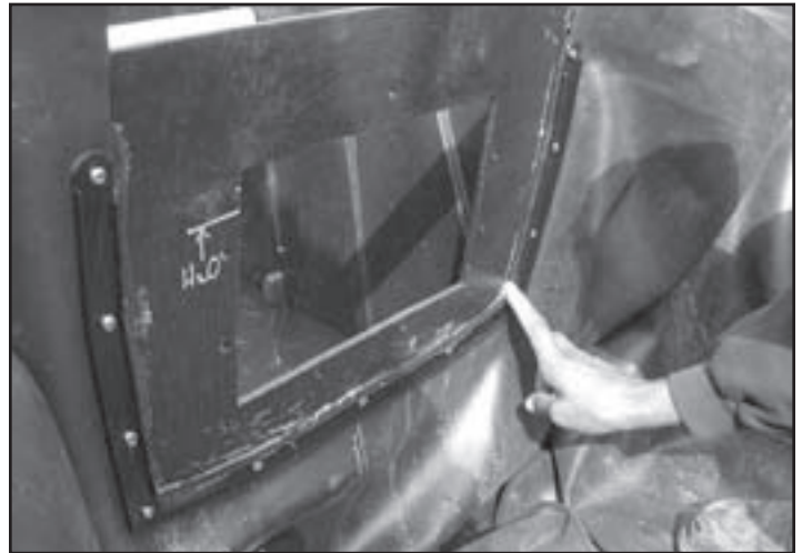
Fig. 18 Apply a 2nd bead of silicone to the inside edge of frame and smooth out with your finger.
