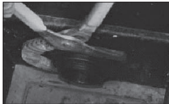
Fig. 2 Attach bulkhead fitting.
