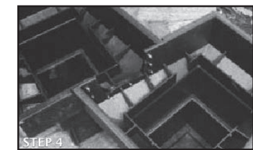
Fig. 8 Bolt vaults together using stainless steel bolts, nuts and washers.
