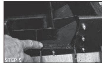
STEP 5 Fig. 9 Apply silicon to vault seams.
