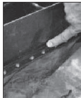
STEP 12 Fig. 18 Apply additional silicone along the cut edge of the liner to create a second seal.
