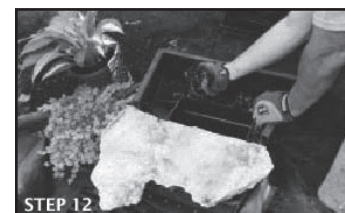
STEP 12 Fig. 19 Apply black waterfall foam under the waterfall stone.
