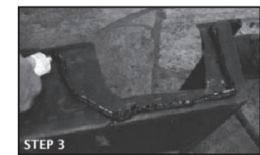
Fig. 7 Apply a thick bead of silicone.
