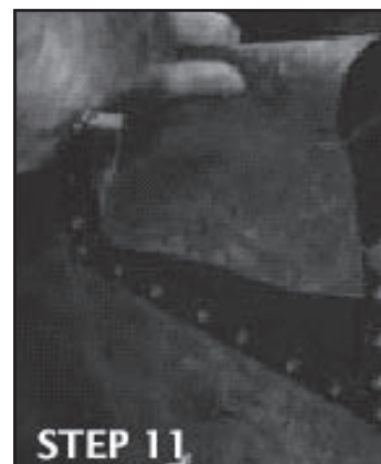
STEP 11 Fig. 17 Trim the liner above and immediately adjacent to the liner attachment strips.
