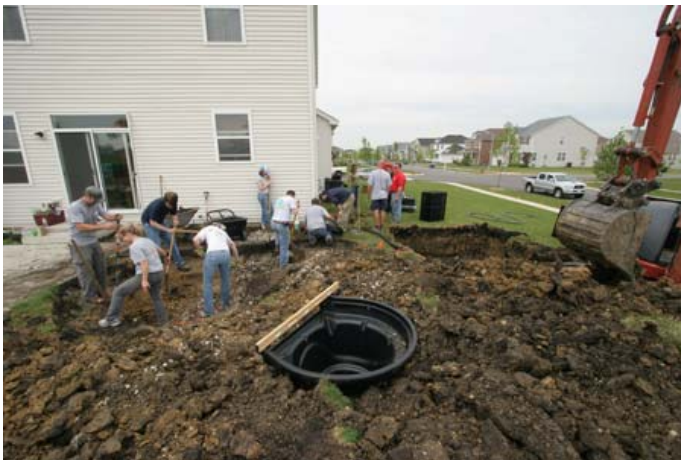
Excavation of site. Rainwater storage basin in background and BioFalls® Filter shown in foreground where waterfall will begin.
