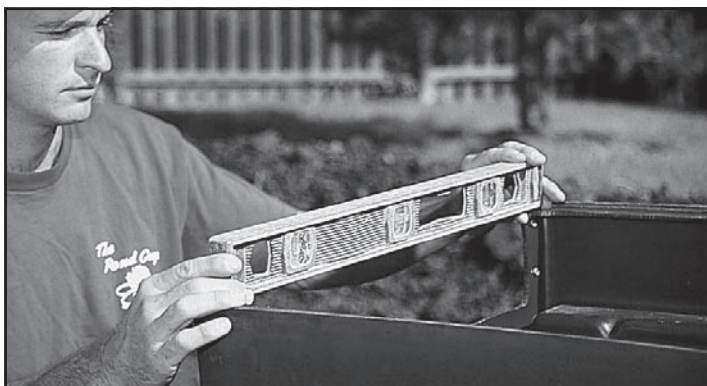
Fig. 3 Level the BIOFALLS® filter side to side as well as front to back.
