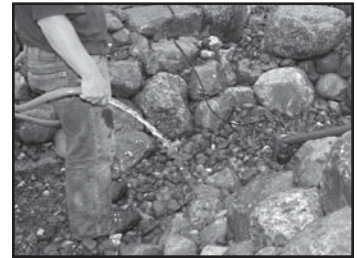
Fig. 22 Set larger boulders (6" – 18") around the perimeter of the basin.
