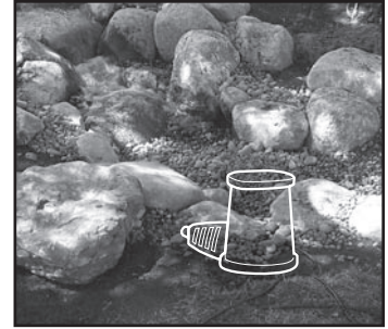
Fig. 22 Set larger boulders (6" – 18") around the perimeter of the basin.
