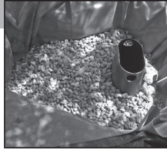
Fig. 21 Add the 1 1/2" to 2" size gravel.
