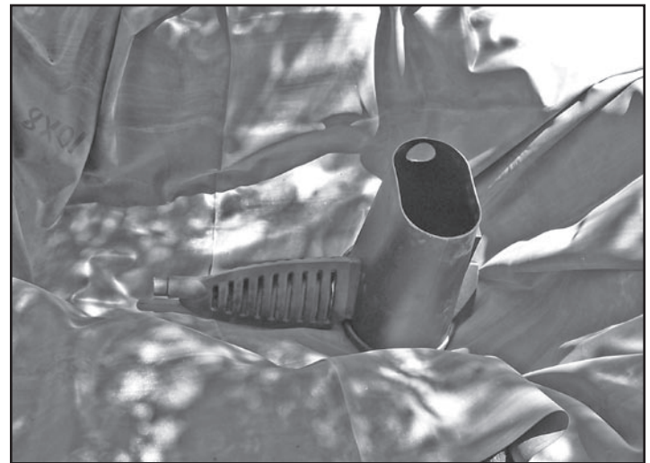
Fig. 7 Place the MicroSnorkel™ Vault and MicroCentipede™ Module on top of the liner.
