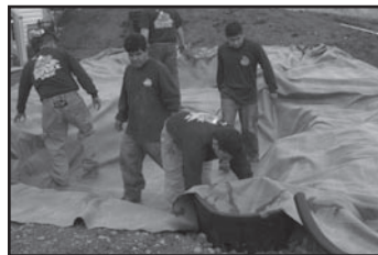
Fig. 6 Place the liner on top of the underlayment following the same installation procedures.
